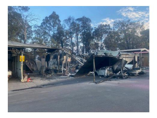
The damage to the Timber Treaters business did trigger a HAZMAT incident due to contamination caused by the release of Copper Chrome Arsenate (CCA) from burnt CCA treated logs. An exclusion zone was established and residents requested to evacuate due to health and safety concerns. DFES engaged contractors to stabilize the piles of CCA ash to prevent it spreading.
